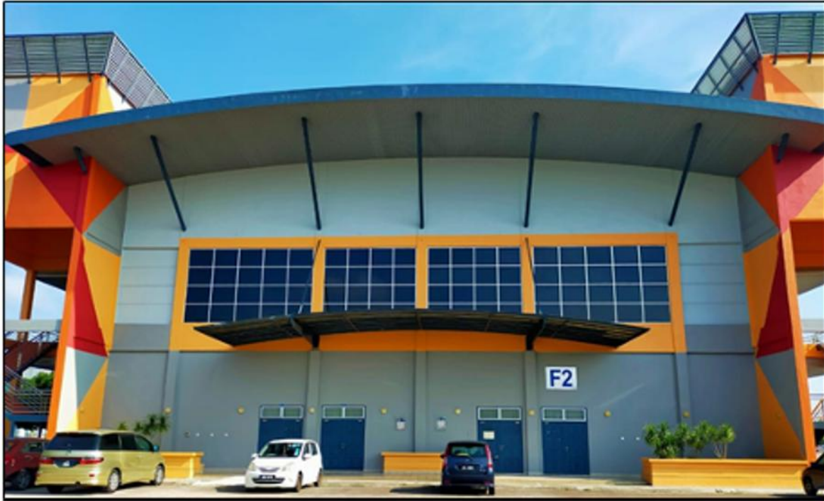
Figure 1. Exterior View of Building F2
